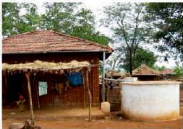
10,000 litre Ferrocement Tank at More wadi, Taluka Karjat Dist. Raigad
