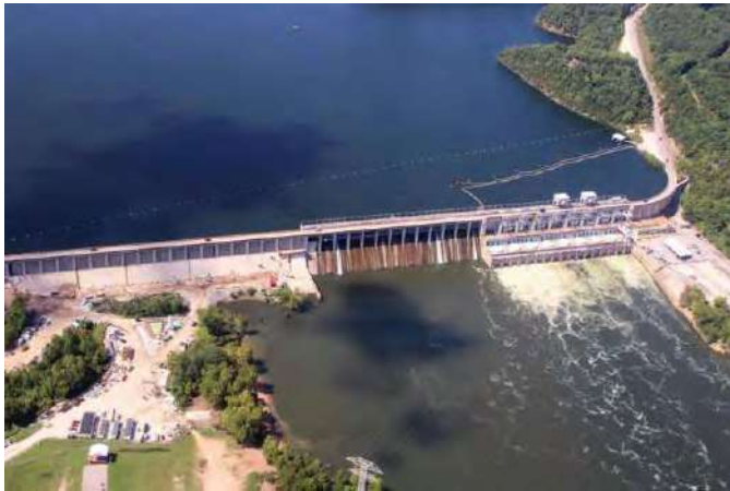
Bagnell Dam is located on the Osage River in Missouri.
