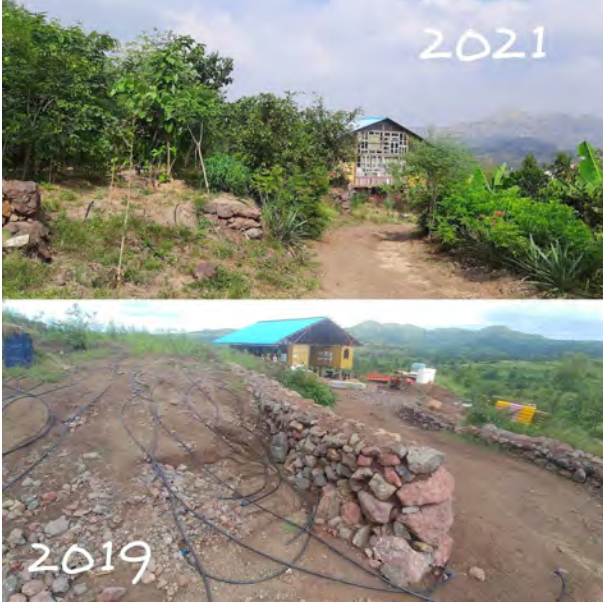
Kamba Farm Structure
