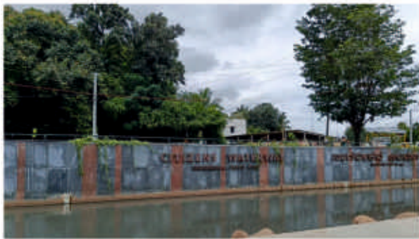
A view of K-100, where the lettering on the wall marks it out as a space to be enjoyed by the public
