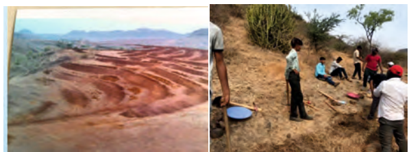
Continuous Contour Trenches (CCT) on foot hills of Pingori
