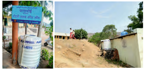
Water Tanks installed for Drinking Water and Toilets at Wagheshwari School at Pingori
