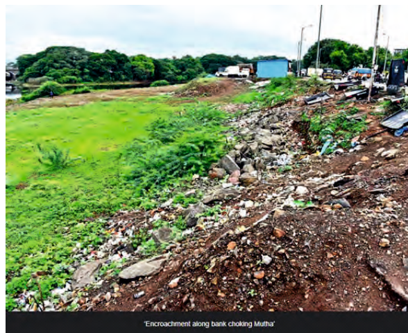
Encroachment along bank choking Mutha
