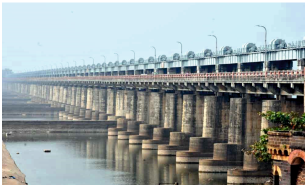
Sir Arthur Cotton Barrage near Rajahmundry in Andhra Pradesh
