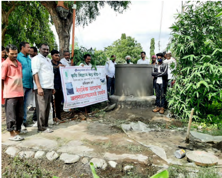
Ferro –Coconut coir Cement Tank above Ground at JSS –Beed to store Water
