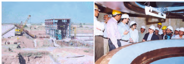
Installation of Siphon at site
