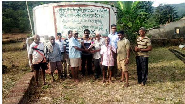
Water scheme at Getachi Wadi , Taluka Khed, Dist Ratnagiri
